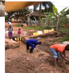
Cleaning of well
