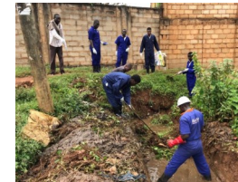
Cleaning of trenches demonstration
